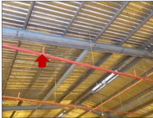
Water Deluge System / Water Spray System
